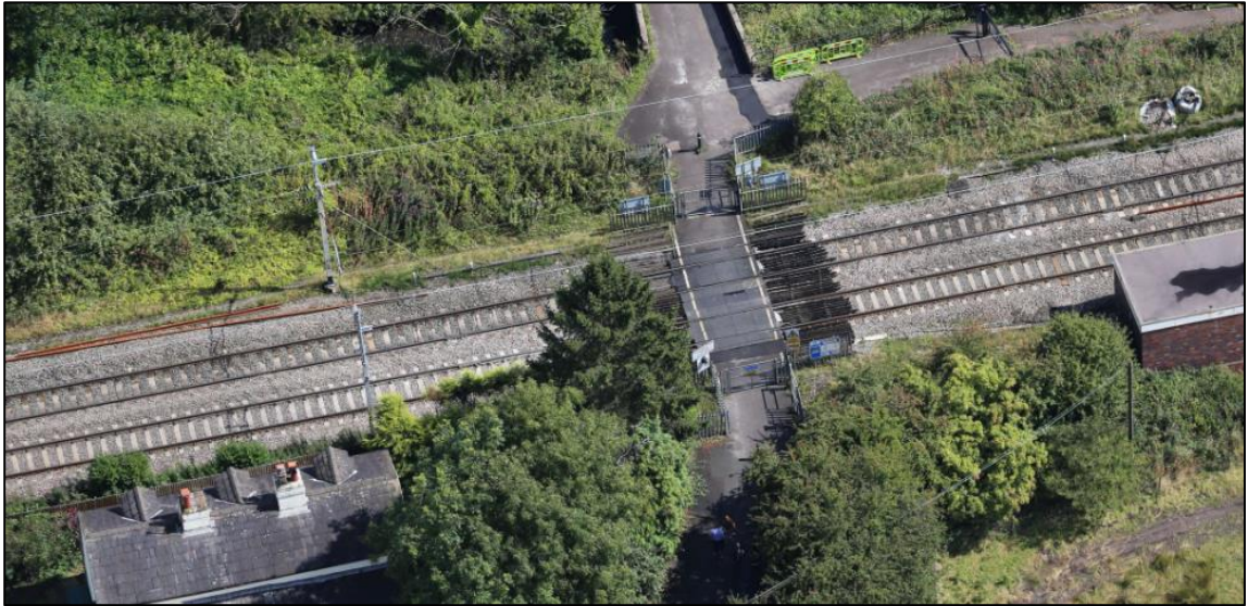
Aerial view of Norton Level Crossing
