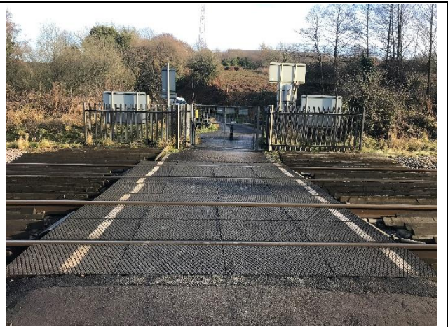
Down side across crossing
