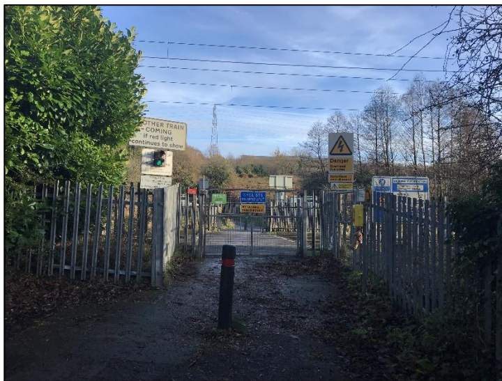
Down side approach of Norton Crossing
